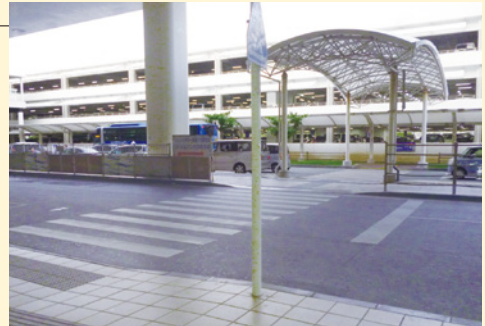
Crosswalk at Gate ④, North side of 1st Floor Domestic Flight Area
